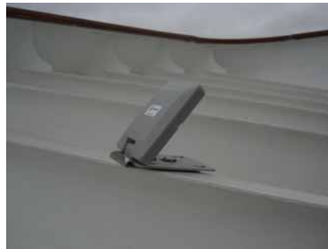
On ship's deck structure
